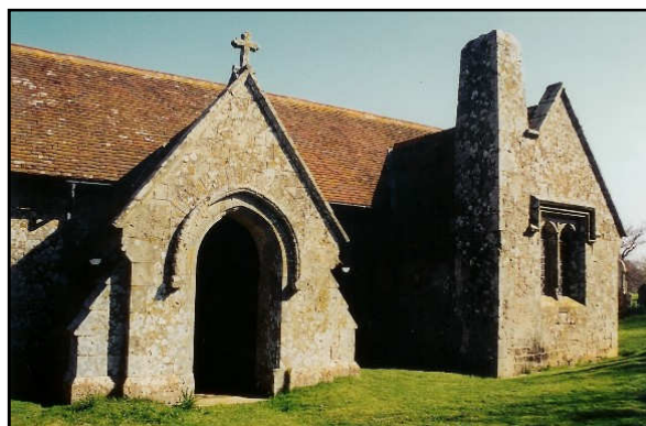
St. James Chapel on the grounds of Kingston Manor.
